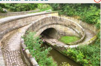
Bridge 77 Lamberts Lane, Macclesfield Canal. This turnover bridge was engineered to allow the horse towing the barge to cross over the bridge without being unhitched.
