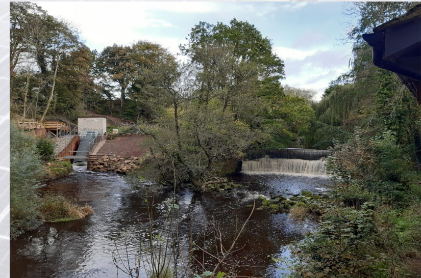
Havannah Weir with the installation complete
