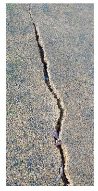
Picture below, taken during the 2017 install, shows the surface of the pathway on which the wet pour surface will be poured. The picture also indicates why the damage to the path surface (reflective cracking) is located in the same place around the circumference of the paddling pool.
