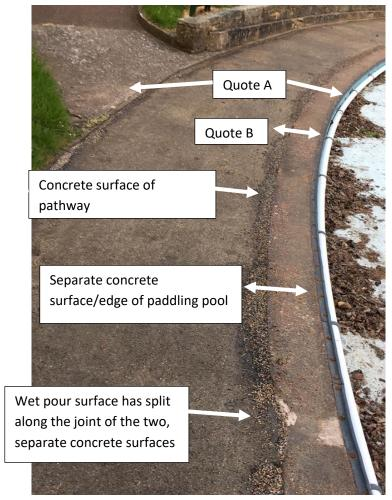
Each company has provided two quotes, Quote 1 to completely replace the wet pour surface over both the pathway surface and the surface/edge of the paddling pool, and Quote 2 to cut away the wet pour surface along the joint of the two concrete surfaces and replace wet pour over the surface/edge of paddling pool only.
