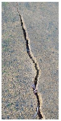
Picture below, taken during the 2017 install, shows the surface of the pathway on which the wet pour surface will be poured. The picture also indicates why the damage to the path surface (reflective cracking) is located in the same place around the circumference of the paddling pool.
