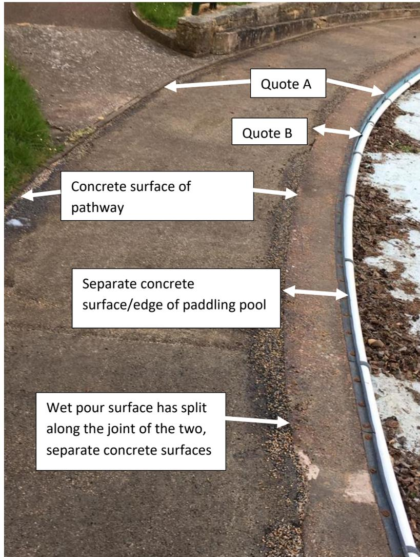
Each company has provided two quotes, Quote A to completely replace the wet pour surface over both the pathway surface and the surface/edge of the paddling pool, and Quote B to cut away the wet pour surface along the joint of the two concrete surfaces and replace wet pour over the surface/edge of paddling pool only.
