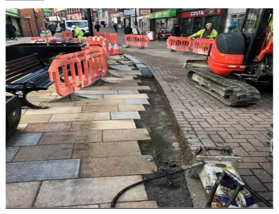
Photo number 2 shows the newly installed keykerbs on Bridge Street (adjacent to Crema Deli).
