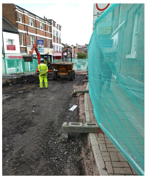
Photo Number 2 shows the removal of the existing carriageway layers at Duke Street.
