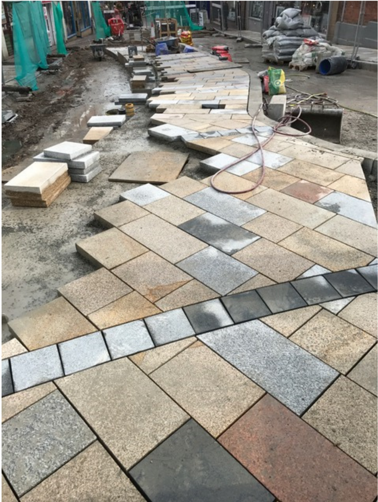
Photo number 3 shows the newly laid section of the north east footway paving at Duke Street.
