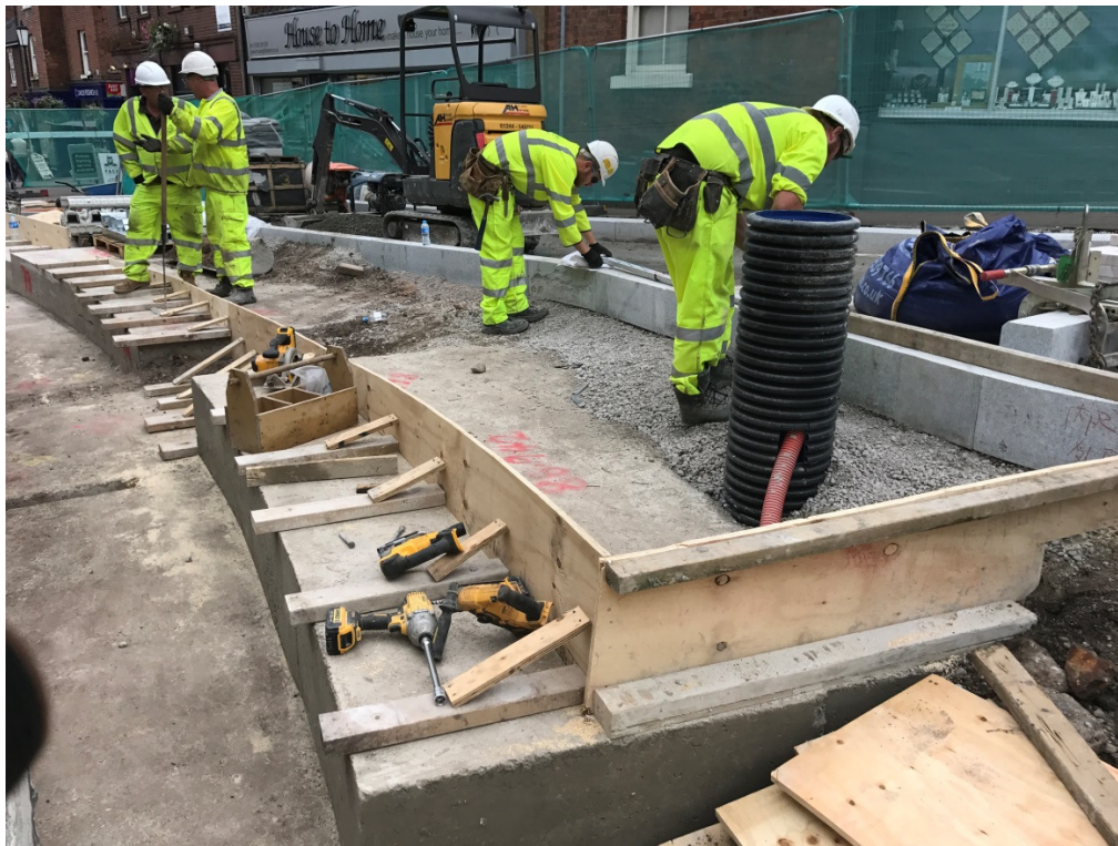
Photo Number 2 shows the installation of the shuttering for the concrete foundation for the granite bench.
