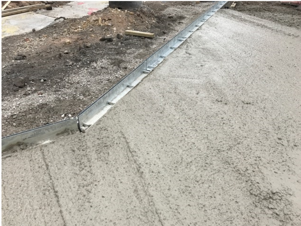
Photo Number 2 shows the installation of the new linear drainage system.
