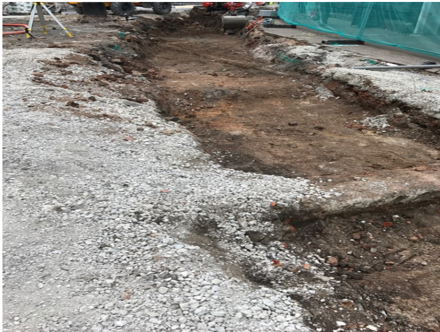
Photo number 3 shows the new granite kerb-line (north section) & the excavated and concreted footway area at Swan Bank.
