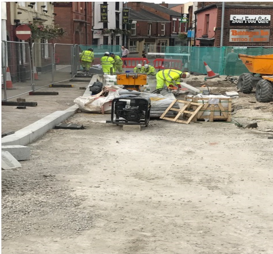
Photo number 3 shows the new granite kerb-line (north section) & the excavated and concreted footway area at Swan Bank.
