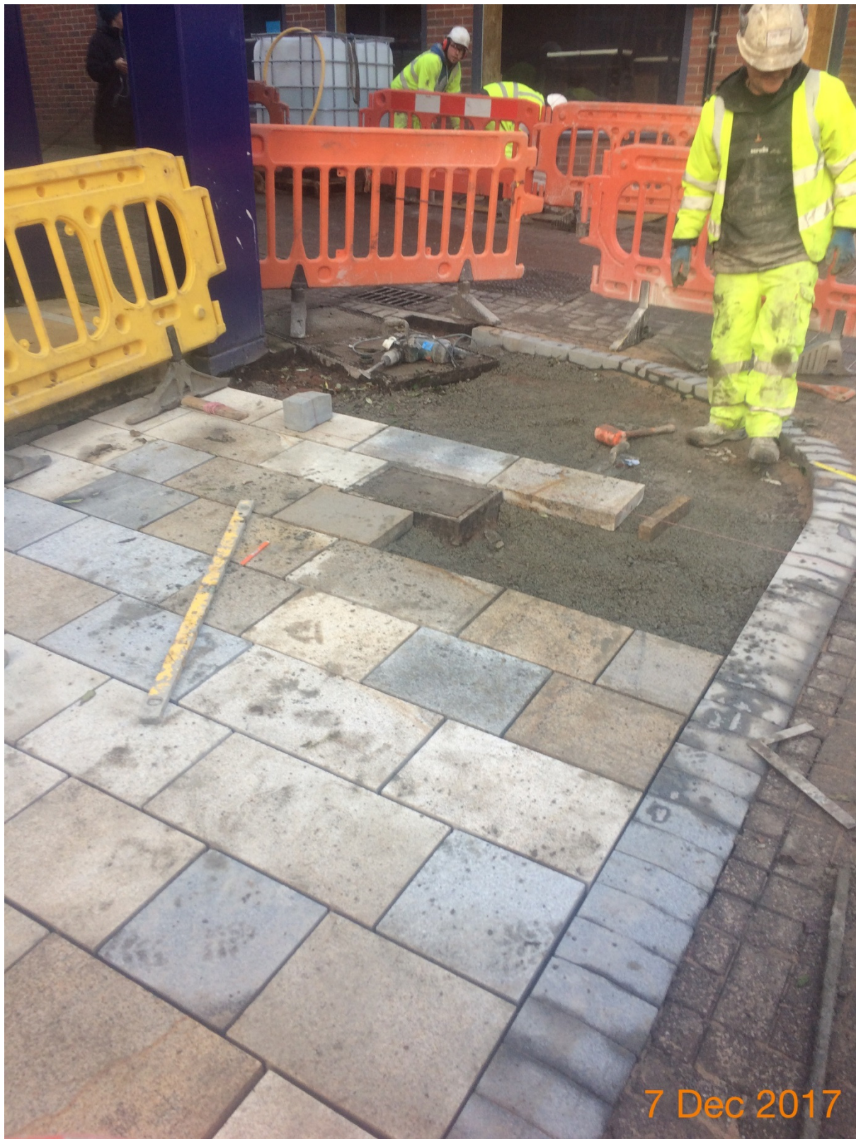
Photo number 2 shows the installation of the new granite block paving on the south footway at Little Street
