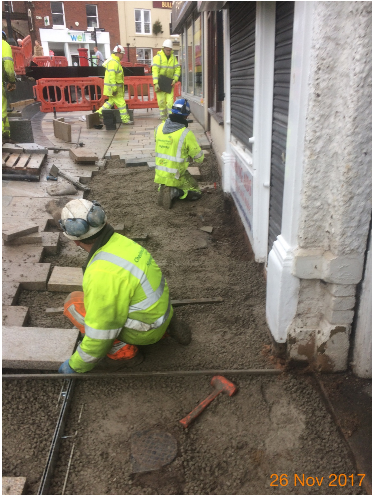
Photo number 3 shows the laying of the new granite paving adjacent to the new granite bench.
