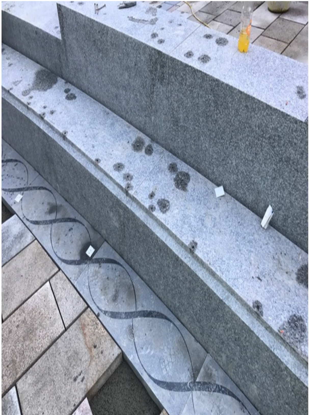
Photo number 4 shows the new ribbon paving adjacent to the bench.
