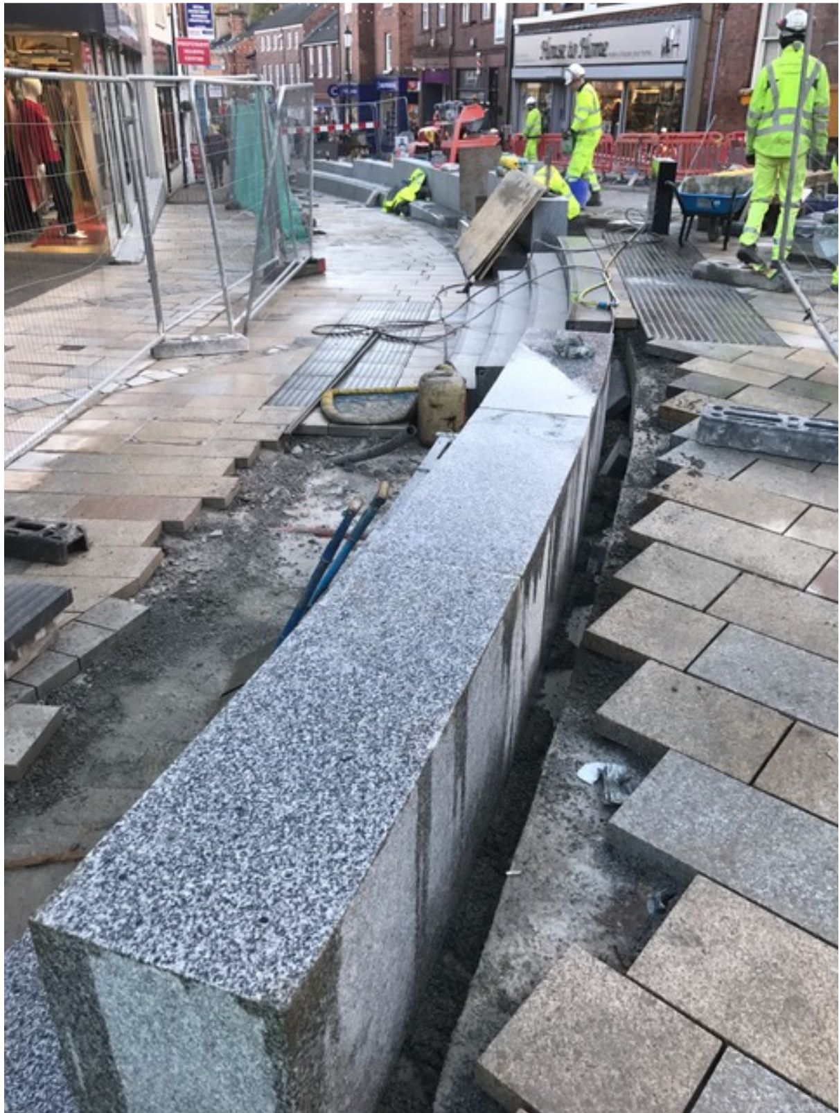
Photo Number 2 shows the newly installed granite bench and steps
