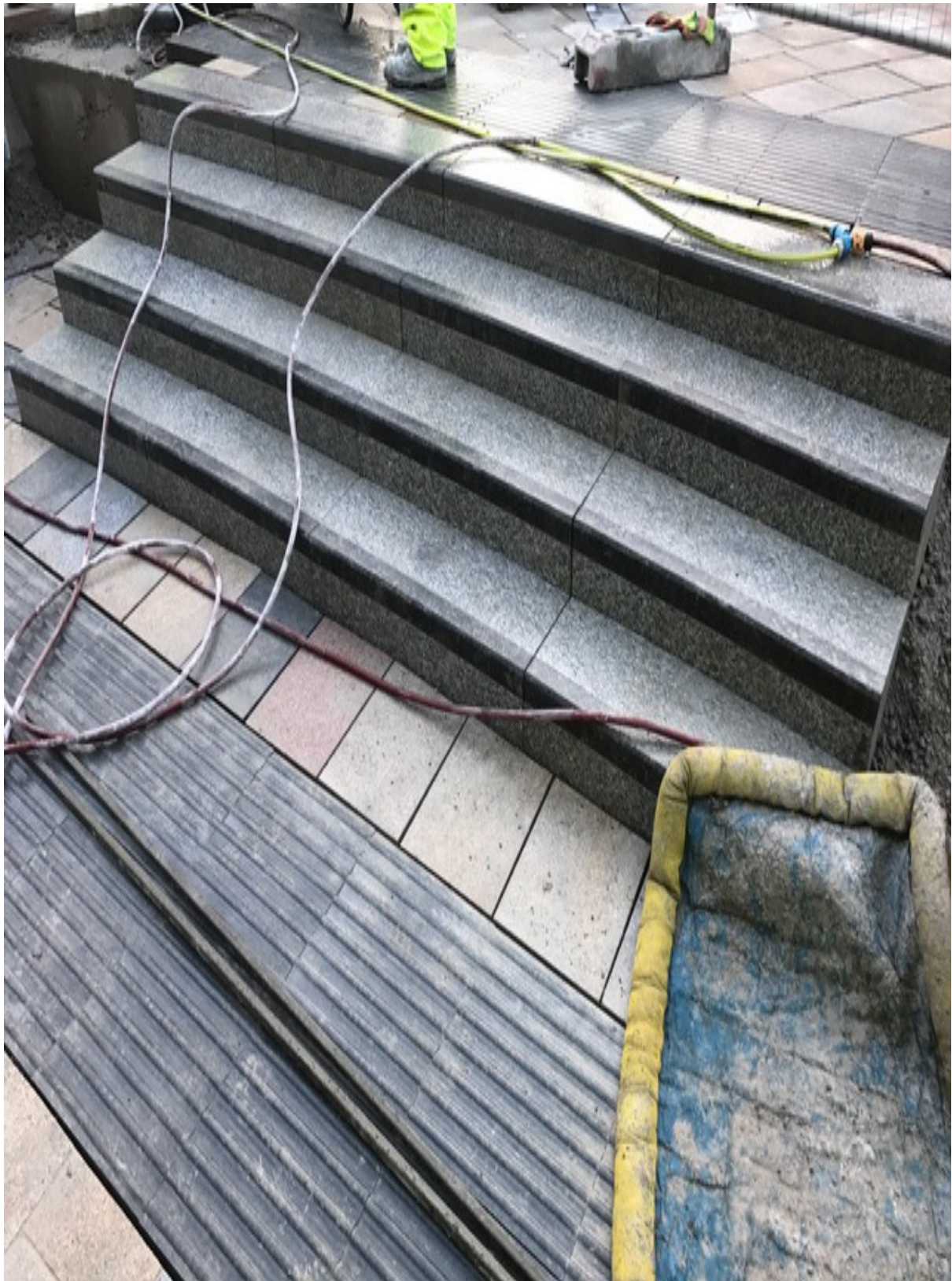
Photo number 3 shows the new granite steps for the new bench.
