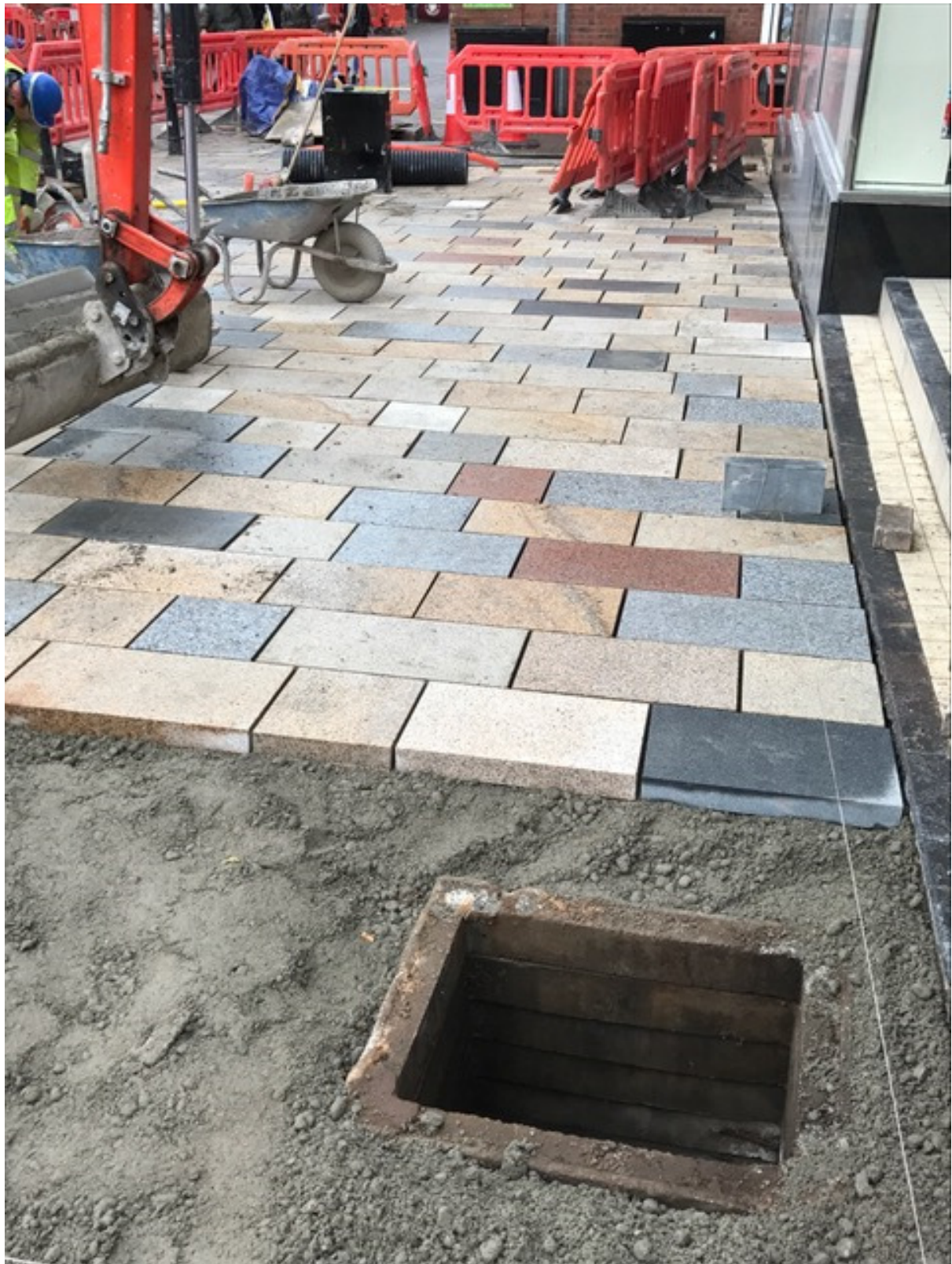
Photo number 3 shows the new granite paving outside of the B & M.
