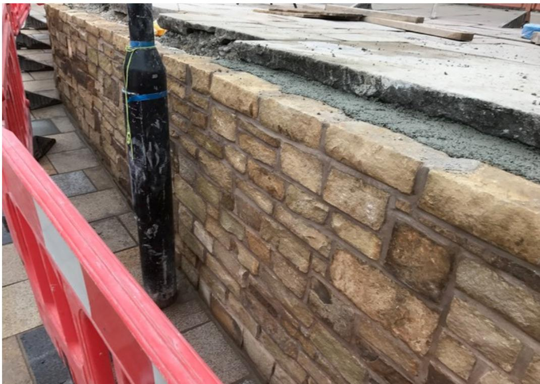
Photo number 4 shows the further construction of the new granite kerbline at the north west footway down to Bridge Street (B&M).
