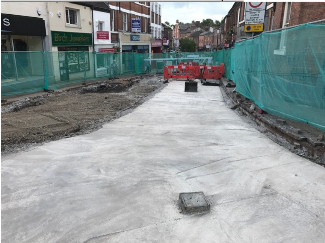
Photo Number 3 shows the excavation for the new footway area
