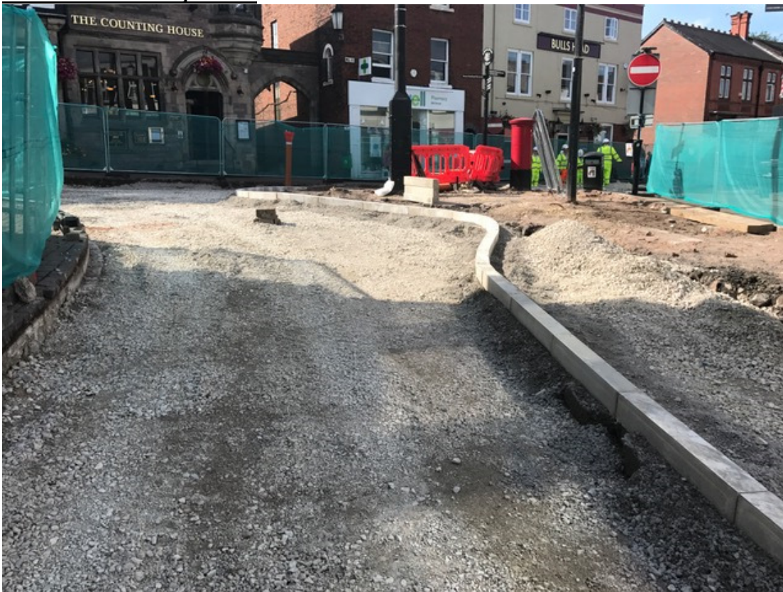
Photo Number 3 shows the construction of the new kerbline and carriageway at the Swan Bank & Duke Street junction
