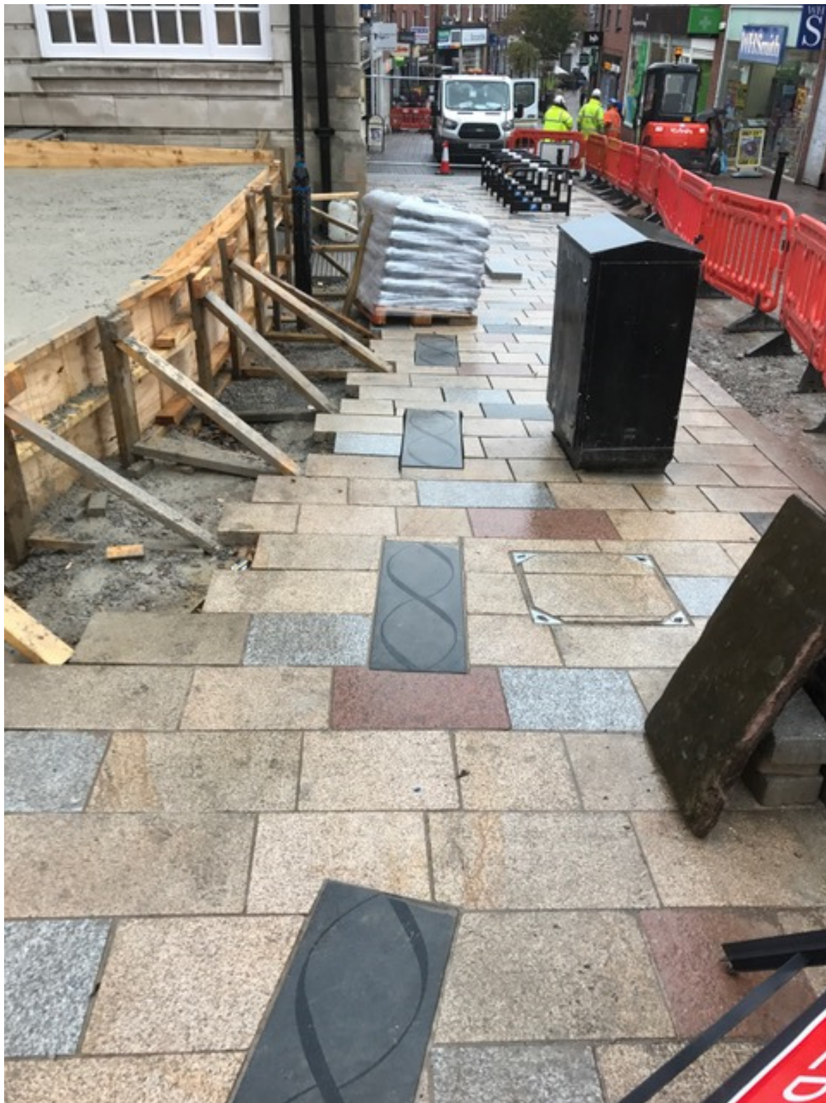
Photo number 3 shows the new granite paving at the south west footway in front of Woolies Wall.
