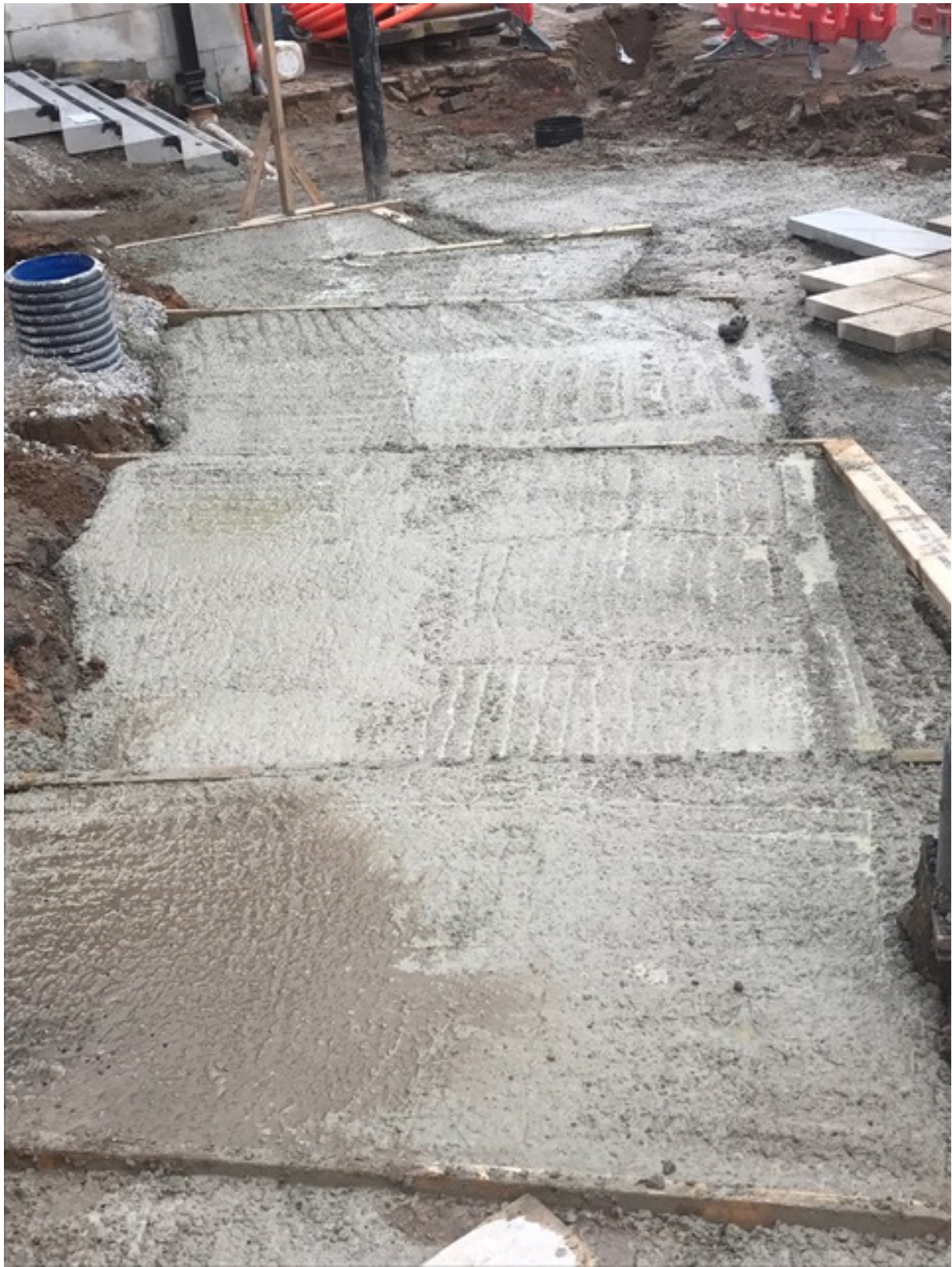
Photo number 3 shows the concrete foundation for the new wall.
