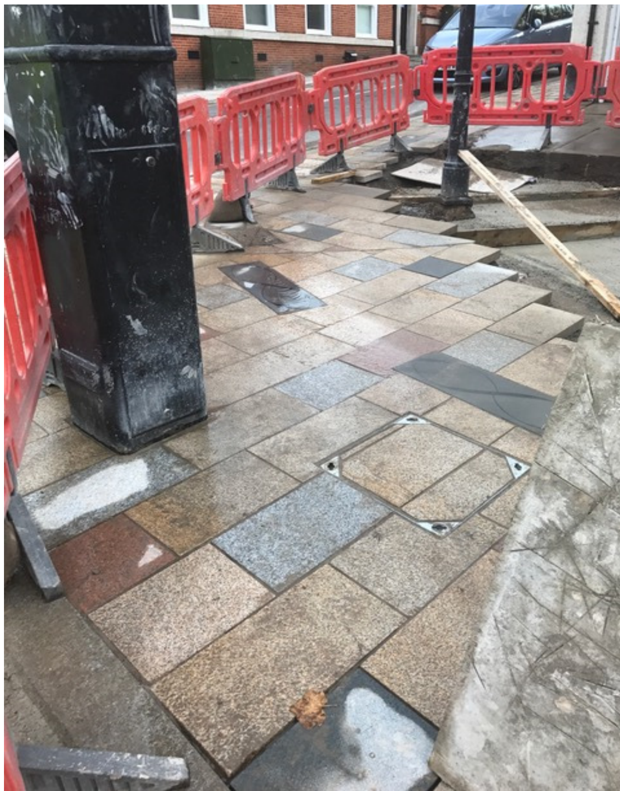
Photo Number 2 shows the new granite paving and kerb-line at the south west footway at Market Street (adjacent to the RBS Bank).
