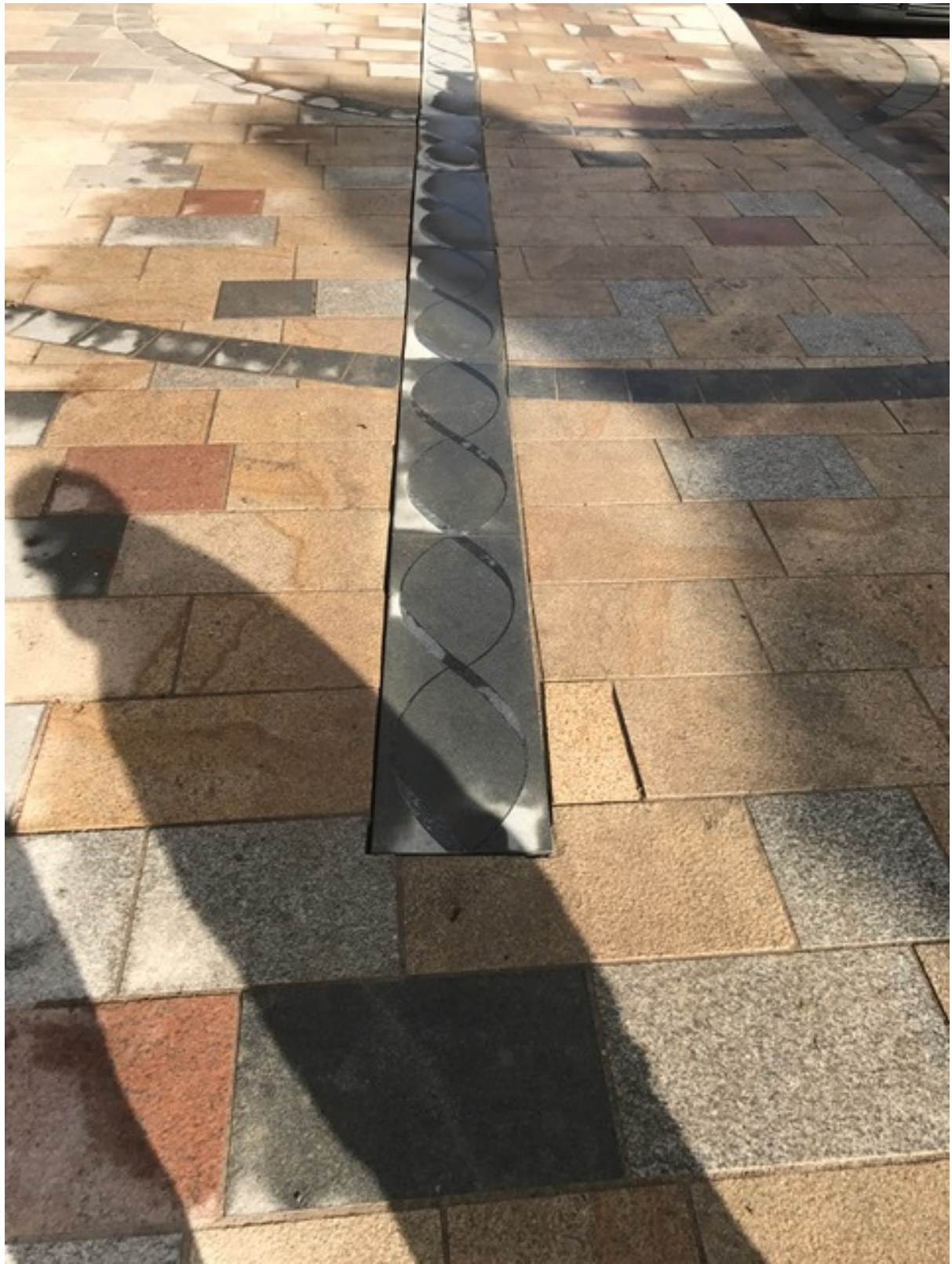
Photo number 3 shows the newly laid section ribbon paving at Swan Bank.
